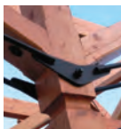
steel brackets, hardware and ties
