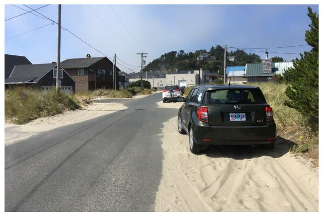
Figure 7: Sand Infiltration on Shore Drive
