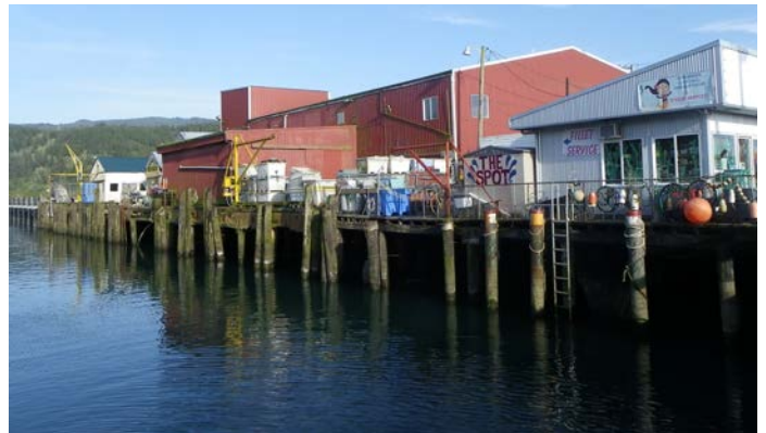
Red building at Port of Garibaldi: seafood processing center
