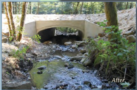
Fan Creek culvert replacement on the upper Nestucca - 2012
